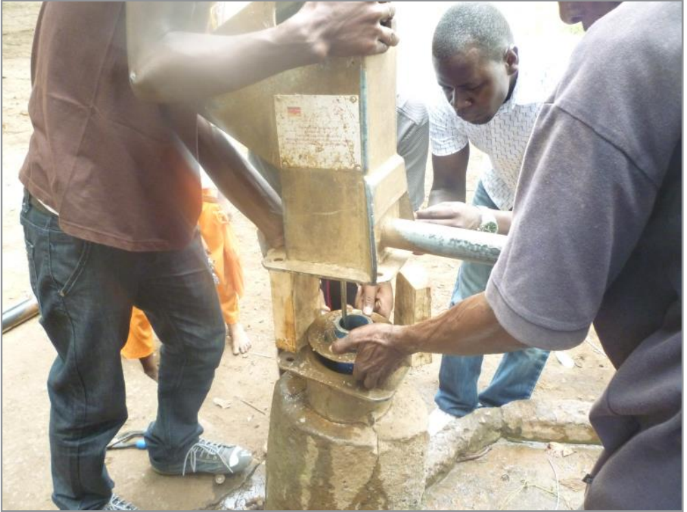
Inspection of hand pump borehole prior to installing water level
