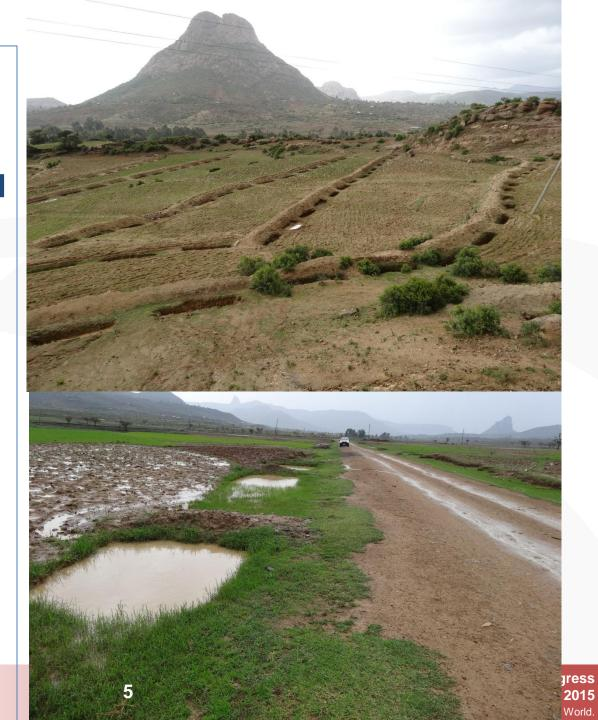
Road side run-off diverted into ponds for surface water storage and groundwater recharge
