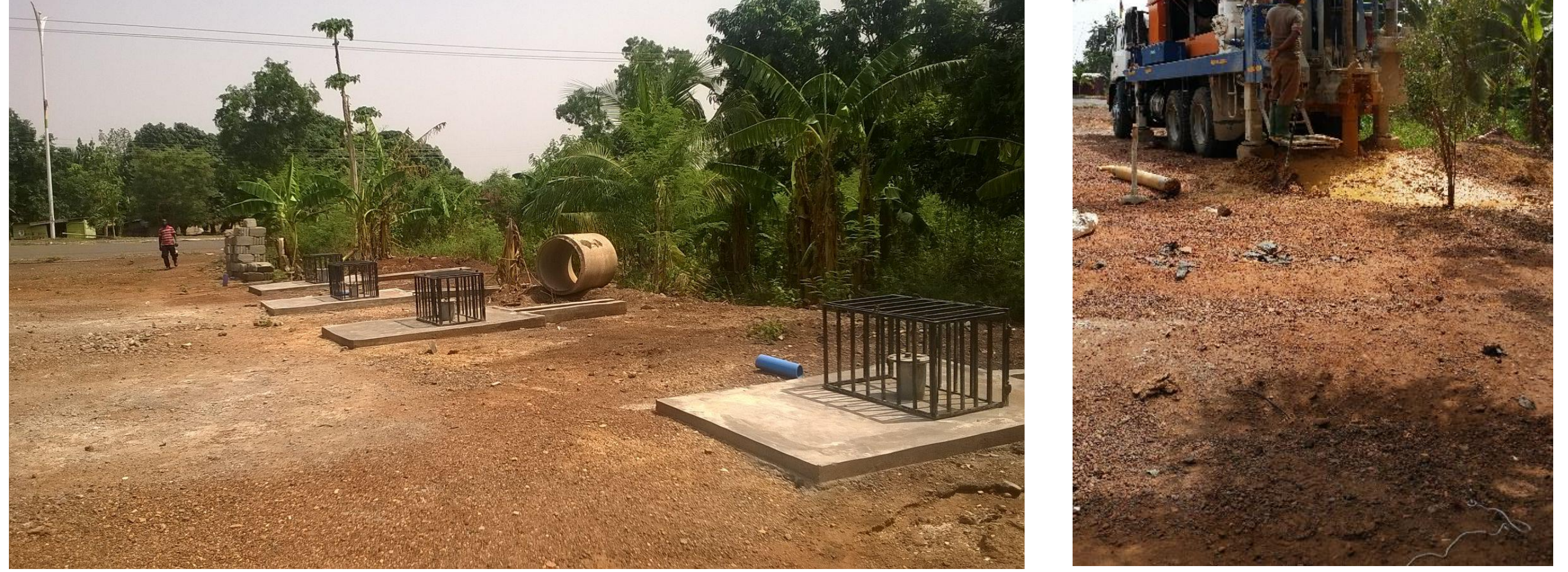
Example of ERT section (upper left); Drilling rig used (right); At bh8, we drilled 4 separate wells of various depths (15, 25, 35, and 50 m; lower left)
