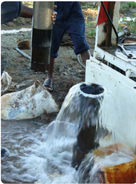
Flowing artesian borehole in Kilimambogo, NE. of Nairobi. Photo by Rotary Clubs of Nairobi, (Kenya), Carlisle, PA and Indianapolis (USA), Edgbaston Convention and Stratford-Upon-Avon, (UK), and Hanau (Germany).
